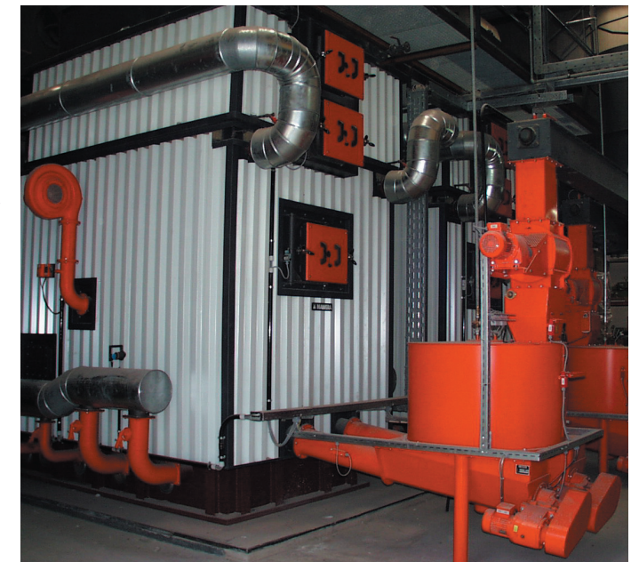
Figure 6: Firebox boiler with a flat moving grate; screw stoker in the front
