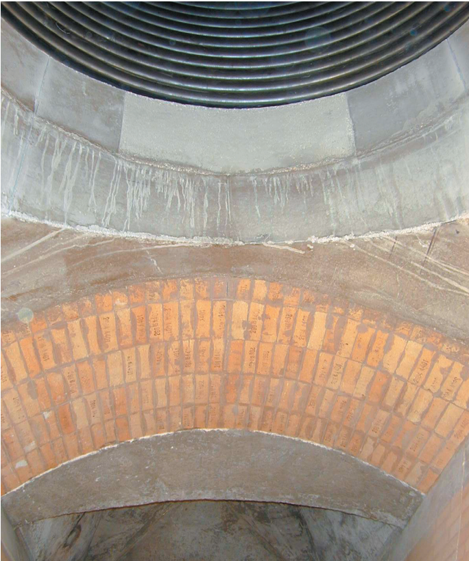
Figure 9: thermal oil boiler adjoining the combustion chamber
