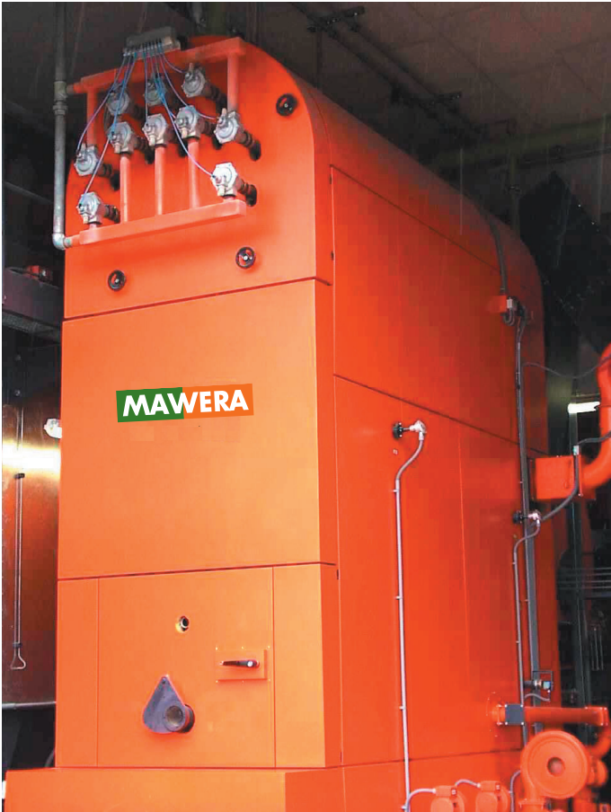
Figure 8: 2.9 MBTU/h MAWERA firebox boiler model FSR 850 Low-NOx with pneumatic boiler pipe cleaning
