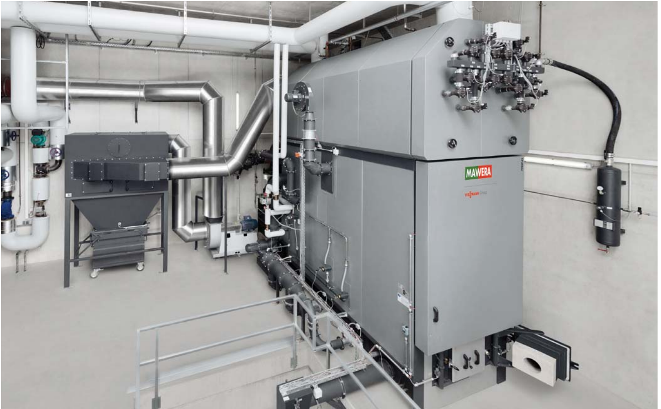
Heating plant at Gräfelfing with Pyroflex biomass boiler
