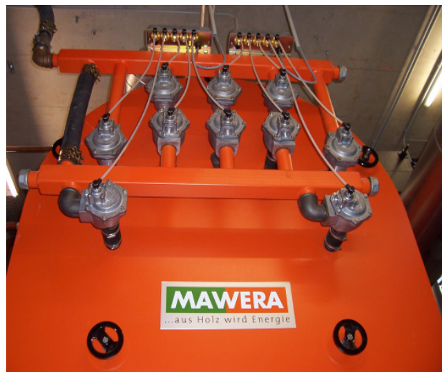
Soot blower for cleaning heat exchanger (optional)
